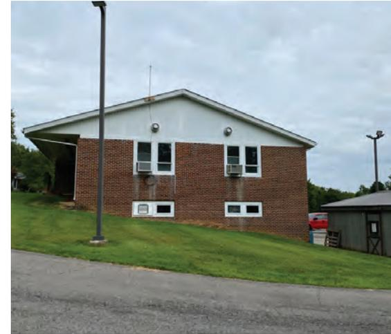
Two rain gardens can be installed on either side of the building to capture, treat, and infiltrate rooftop runoff before it reaches the stormwater sewers. A preliminary soil assessment suggests that more soil testing would be required before determining the soil's suitability for green infrastructure.
